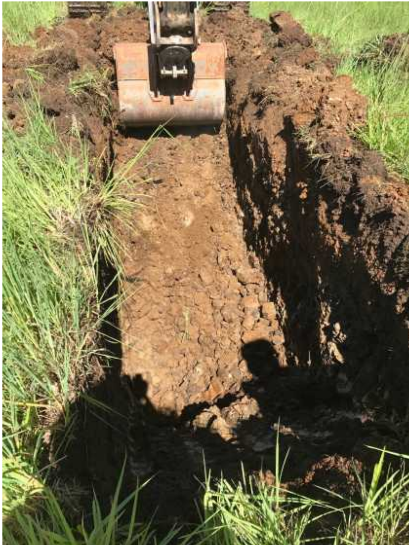
TEST PIT TP13
