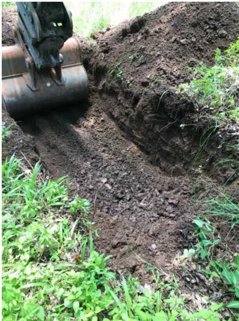
TEST PIT TP4
