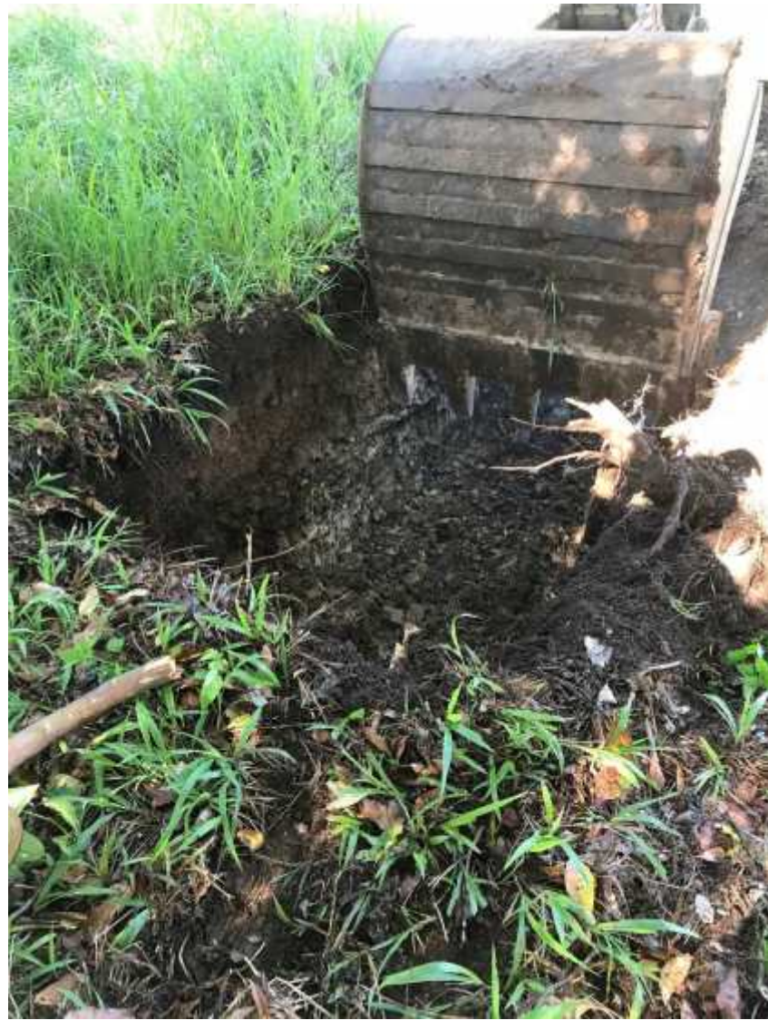
TEST PIT TP10
