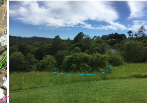
Concave landform possible creep/slumping
