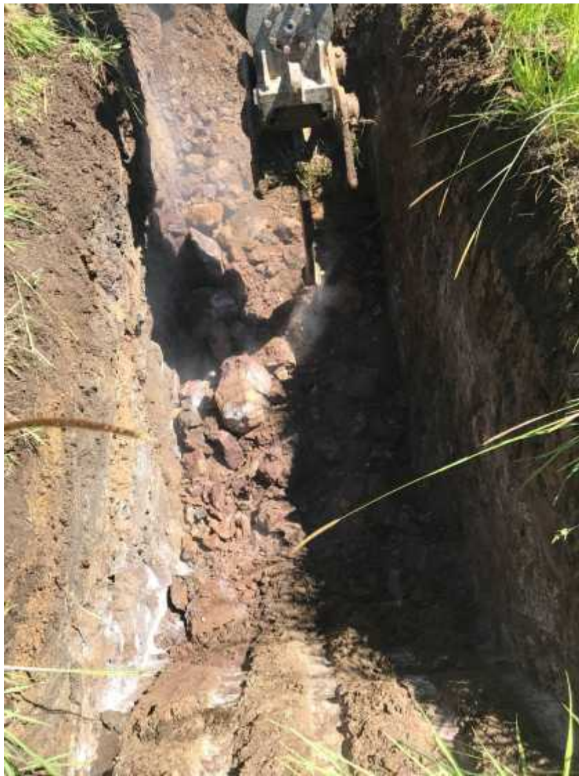
TEST PIT TP11
