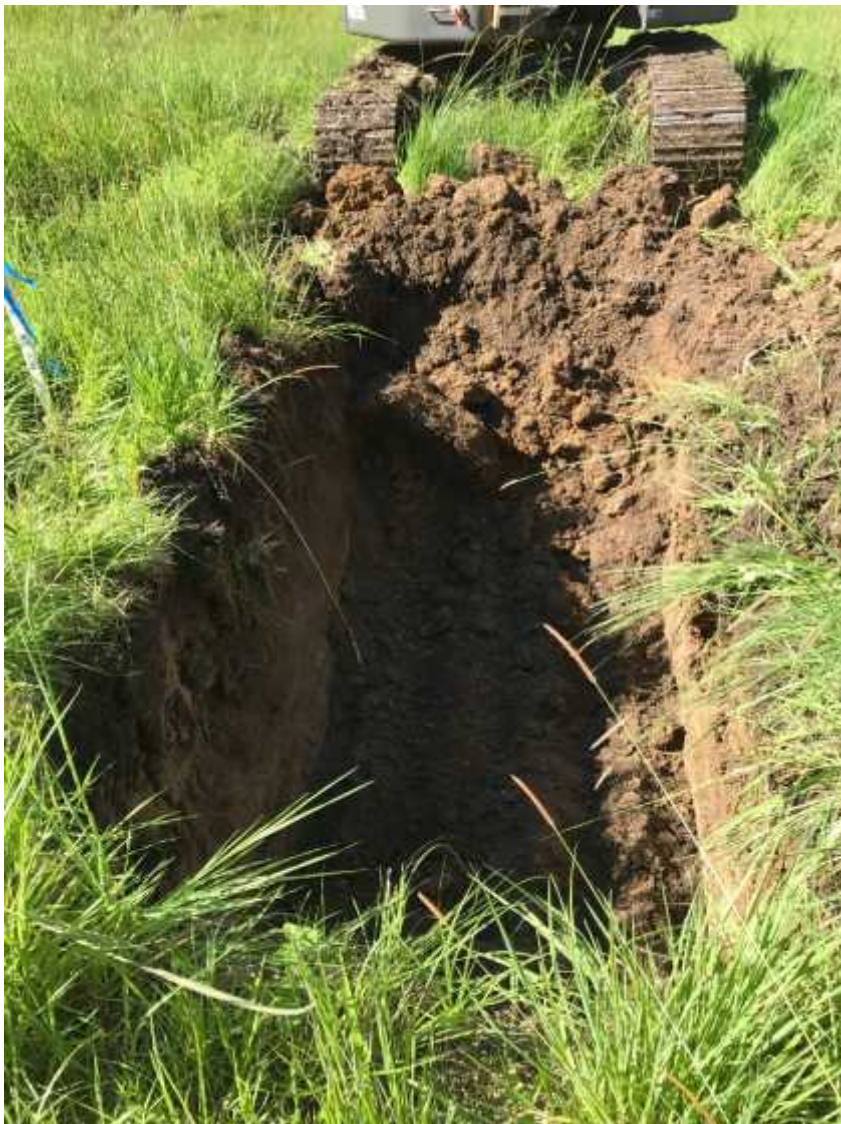
TEST PIT TP6
